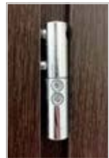
Useful four hinges \varnothing 16 with 3D adjustment
